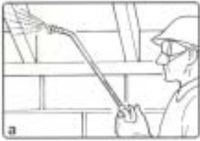
BORA-CARE can be applied: a) in basements and crawlspace; b) on unfinished wood floors; c) in attics; and d) on outdoor wooden structures.
